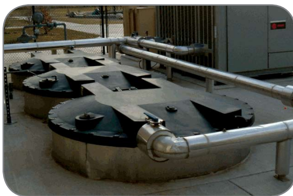
Above: Three Calmac Ice Tanks buried in-ground next to a Trane air cooled chiller. Top right: Large above-ground Calmac Ice Tank Farm served by a Trane water cooled Centravac
