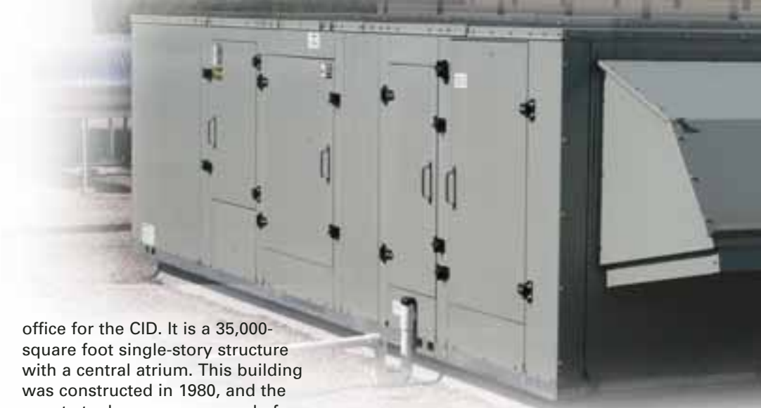
Trane 100 percent fresh air handler, Model FADA, maintains a temperature-neutral discharge-air condition.
