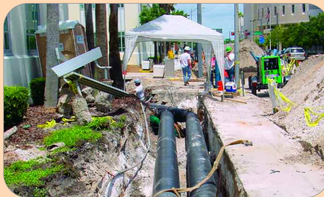
Underground piping in progress.
