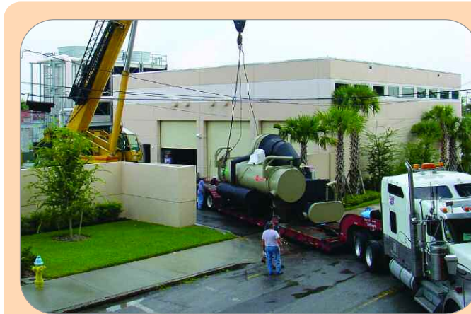
New 1,500 ton Trane Centravac being delivered.
