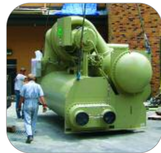
Replacement 1000 ton chiller being rigged into place.
